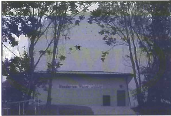
New North Booster Pumping Station at Atkinson Park.
