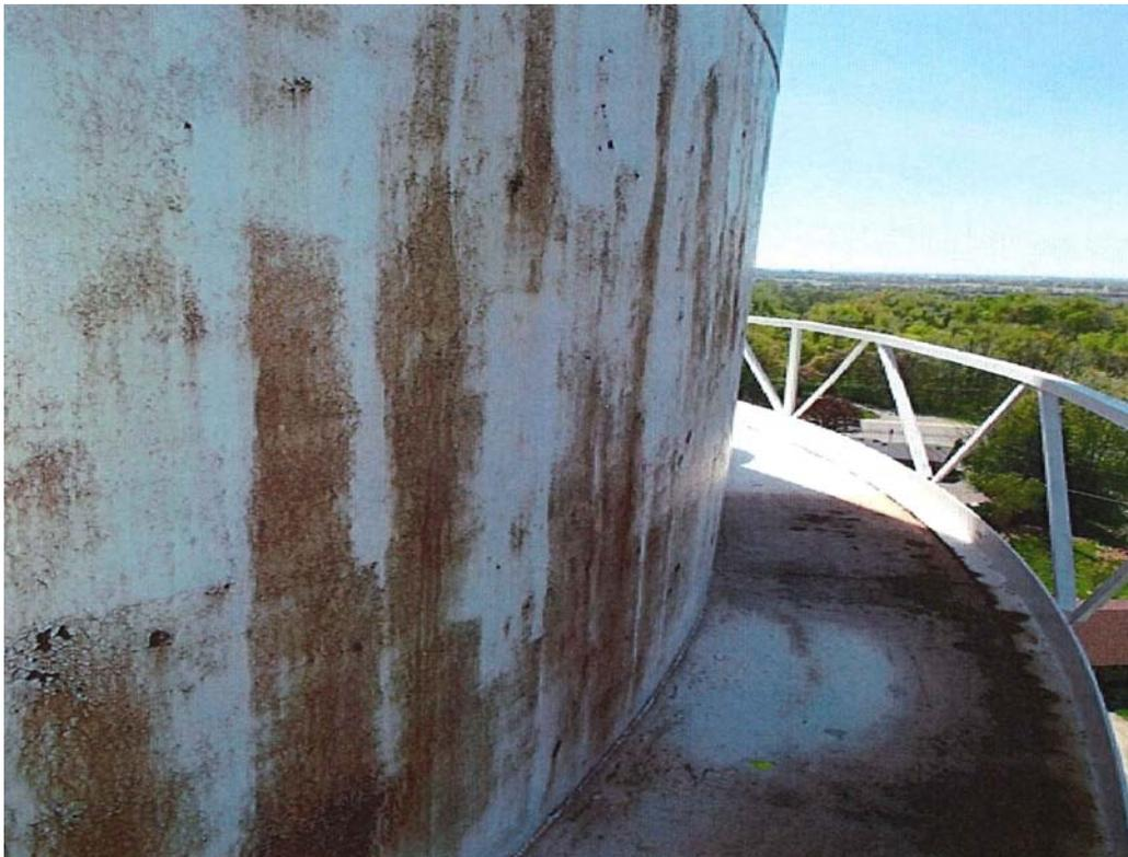
*Corrosion on shell and balcony of the Frontier Tank*
