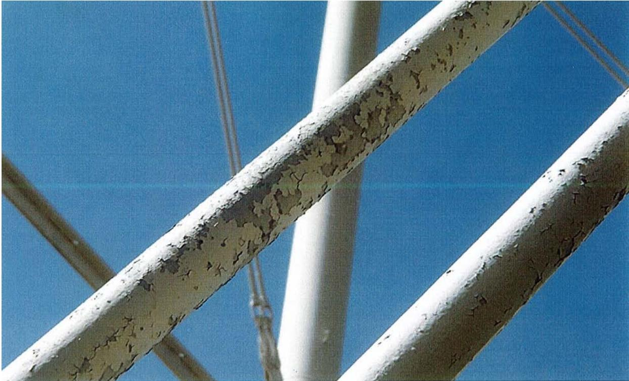
Corrosion on Diagonal Bracing - College Tank
